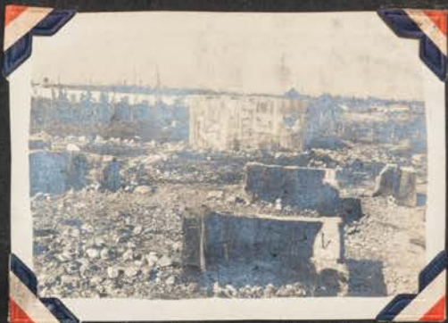
Gas water tanks right off the airfield
