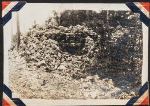
Gas in bunker bunker
